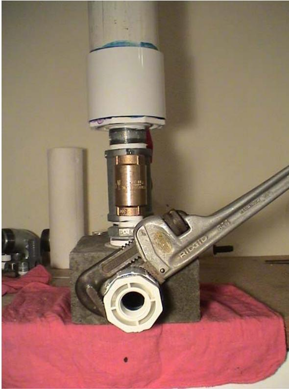
Installing the 2" to 1" PVC Bushing
